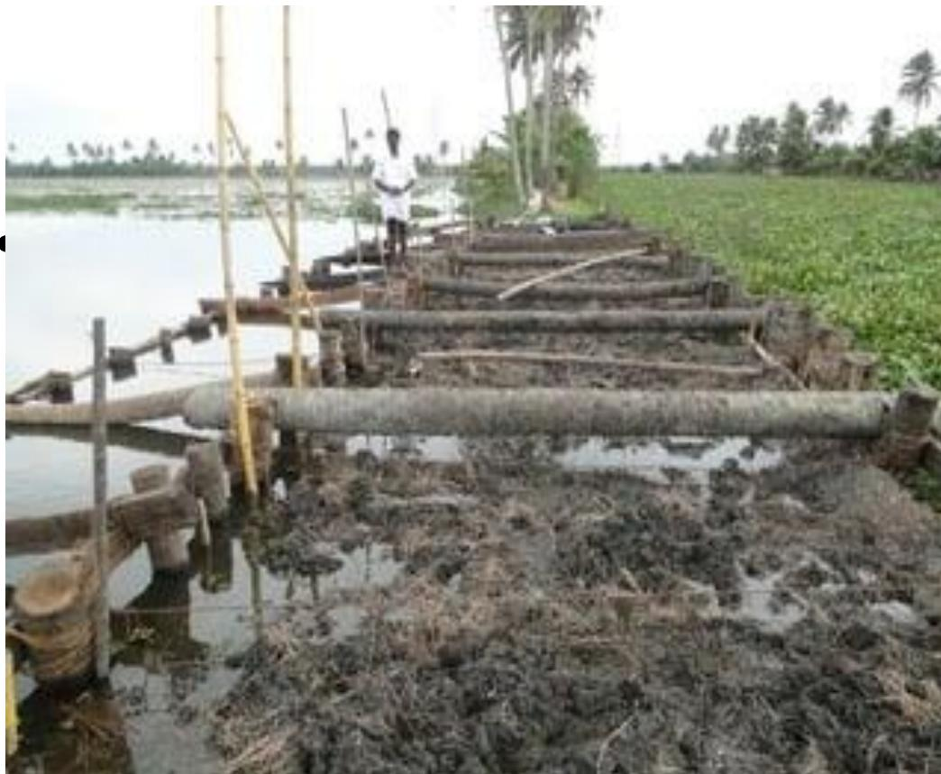
Made of clay, dug out of the canal beds and stabilized with bamboo and coconut trunks on the sides
